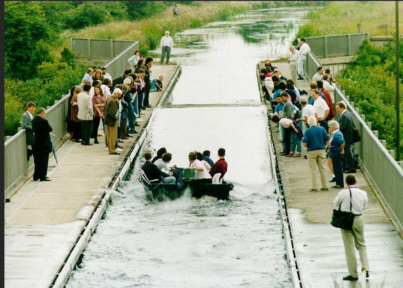
Scott Russell Aqueduct
